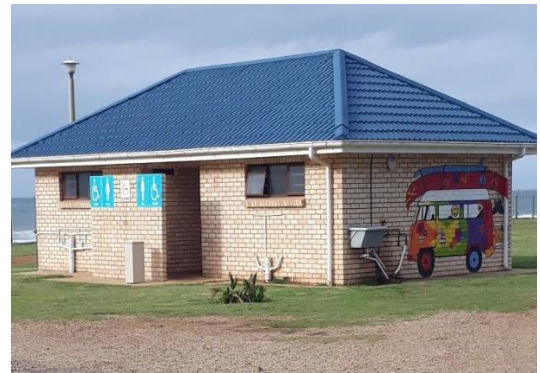
Jeffreys Bay Caravan Park ablution for disabled
