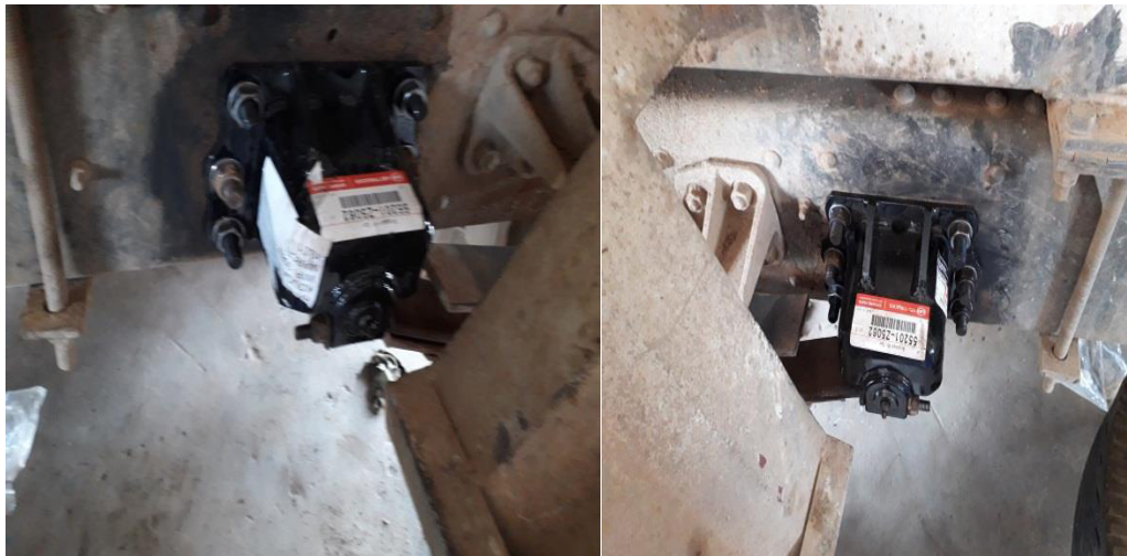
Installing shackle pins and hangers.
