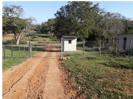
Fencing of Yellow Woods Park and painting of ablution facilities
