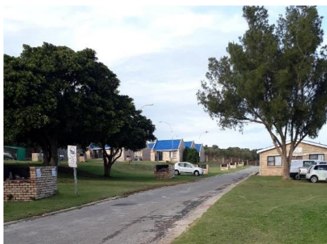
Fencing, painting and repair braai's Pellsrus caravan park
