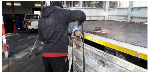
All types of welding work is done in the workshop.
