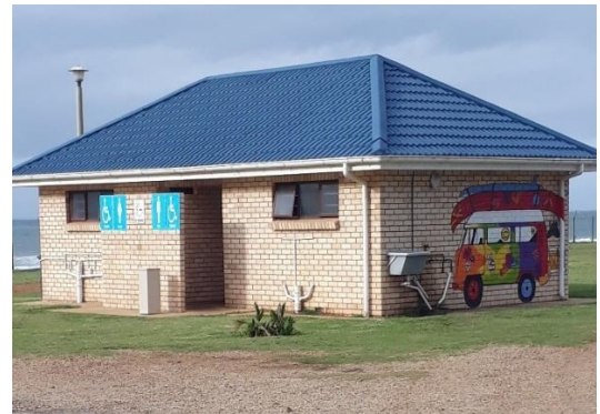
Jeffreys Bay Caravan Park ablution for disabled
