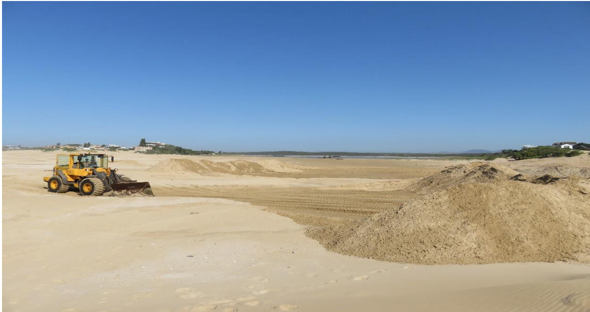
Fig 4. Skimming the dune-sand across the beach adjacent to the sea. The two excavators shown in Fig 3 are seen in the distance. Paradise Beach is on the left of the picture.
