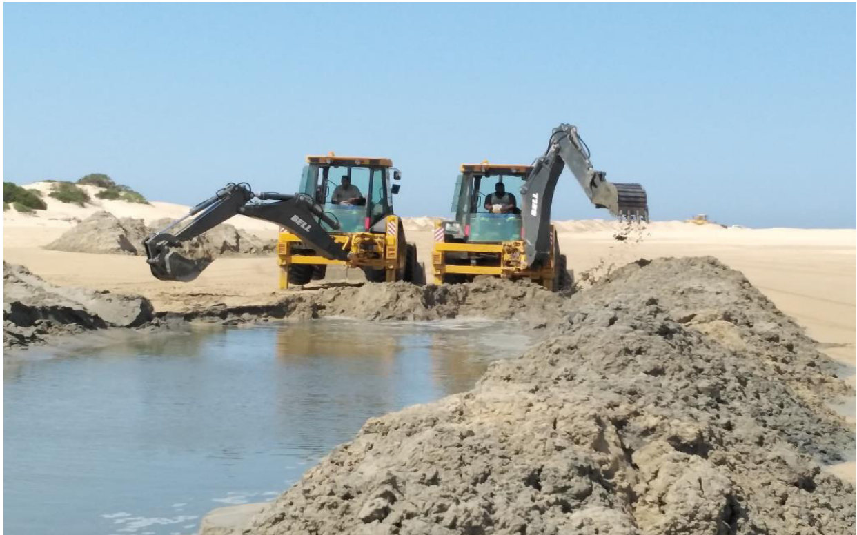
Fig. 3. Excavation of a channel across the 450 m berm on the norther side ( adjacent to the estuary). The channel was about 7 m wide and excavated to a depth of 30-40 cm below the water surface. This channel would link with the beach excavated channel seen in the background.
