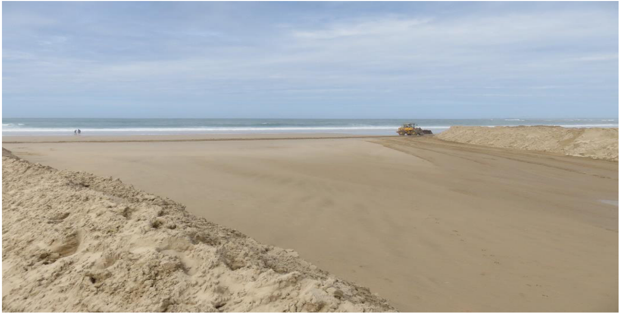
Fig 8. Following a high tide, the entrance to the channel was again skimmed aimed at regulating the inflow of seawater on the following high tide. A total of nine regulated inflows occurred (Sunday afternoon high tide to Thursday 12 March afternoon high). Max tidal height over the period was predicted to be around 2 m.
