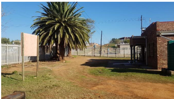
Figure 5: Completion of fencing at Hankey Fire Station
