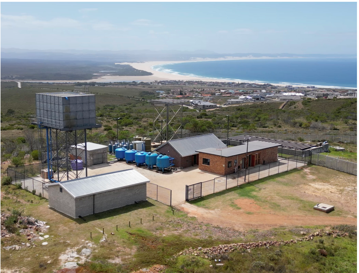
The newly erected water purification plant in Jeffreys Bay – one of four purification plants across the region – purifies transforms 3 million liters of borehole water per day, with the potential to double this output to 6 million liters per day.
