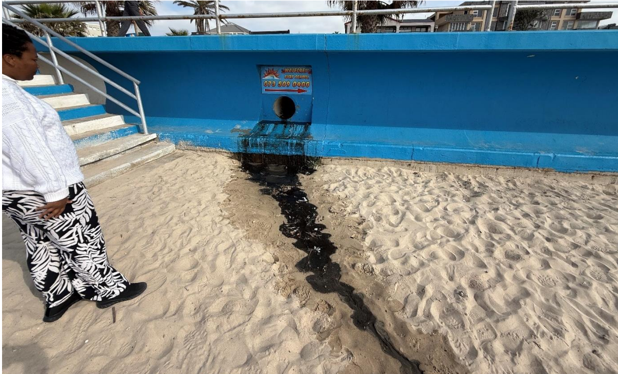
Figure 4.29: A stormwater discharge onto Jeffreys Bay main beach
