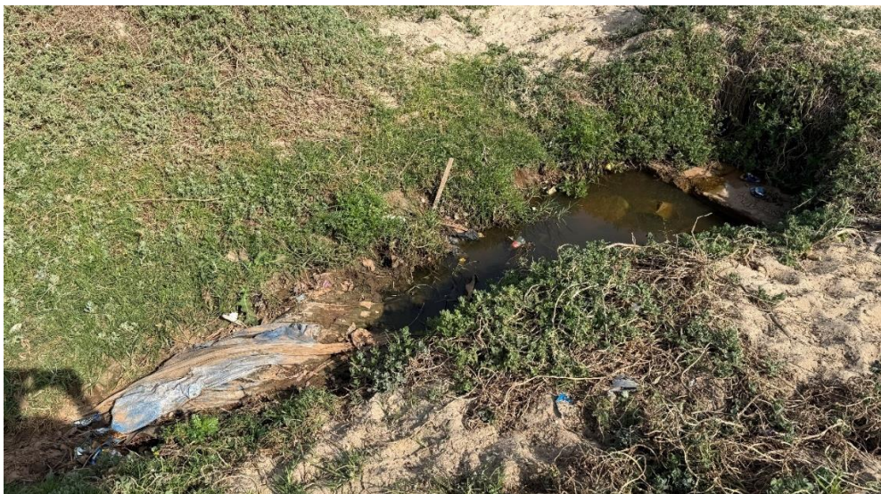
Figure 4.28: Sewerage seeping into the coastal zone along the Jeffreys Bay beach
