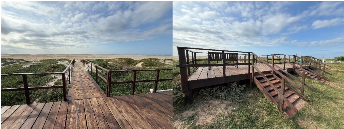
Figure 4.2: Hardened boardwalks at Kabeljous Beach
