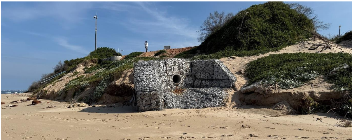
Figure 4.30: Stormwater infrastructure located along Paradise Beach
