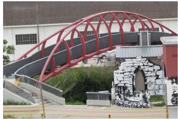
Example of Sculptural Pedestrian Bridge in NMBM (Source: MBDA)
