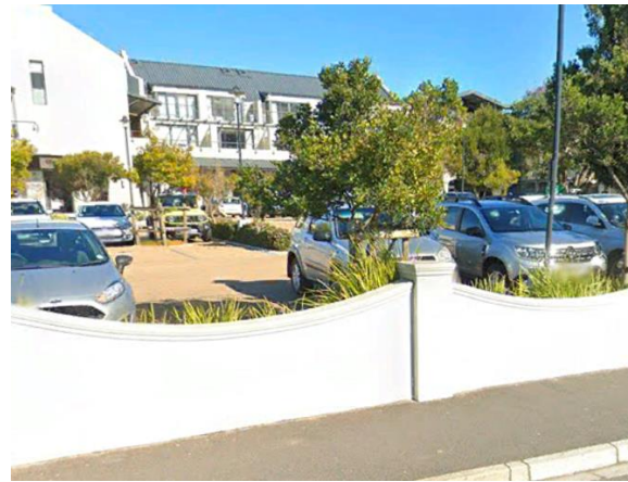
Parking shielded by low white walls (Hermanus) (Source: Google Earth)
