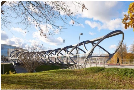
Example of Sculptural Pedestrian Bridge (Source: ArchDaily)
