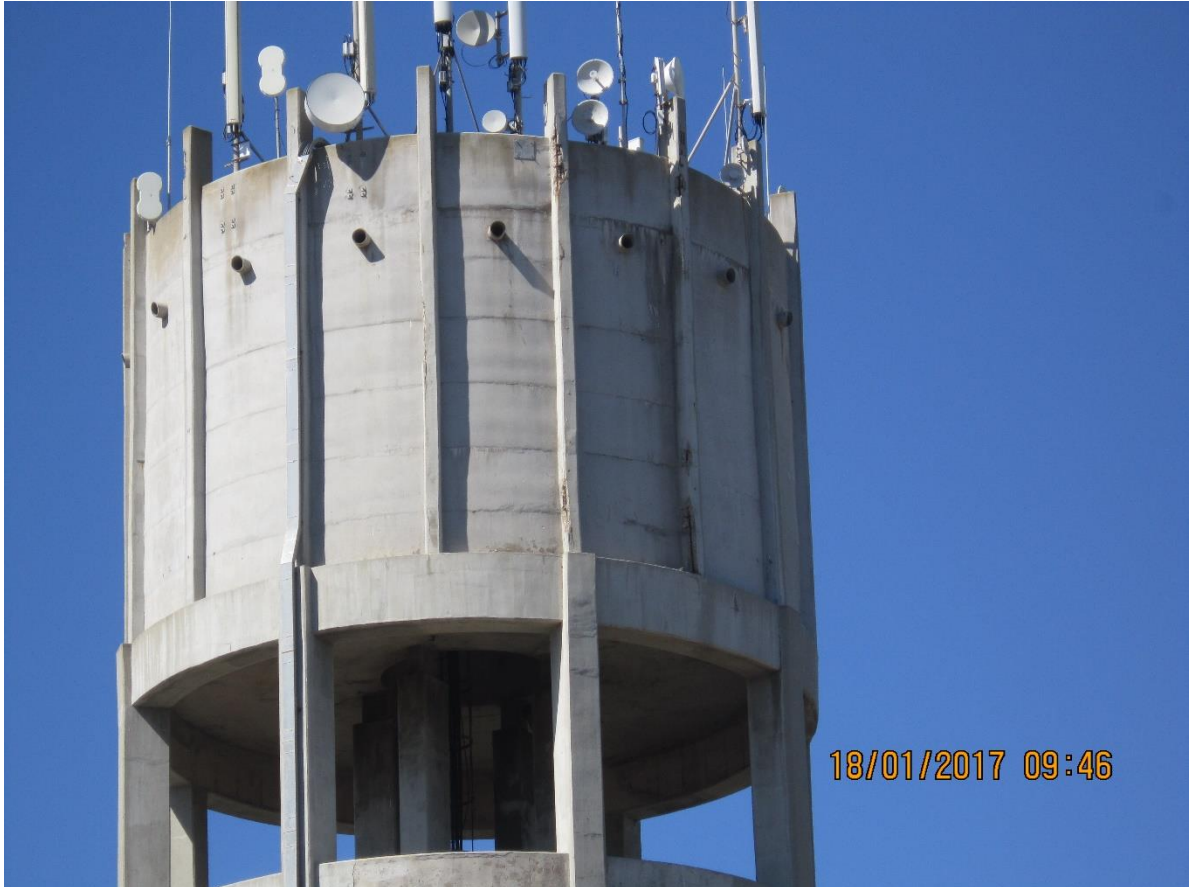
Figure 3: Paradise Beach Water Tower
