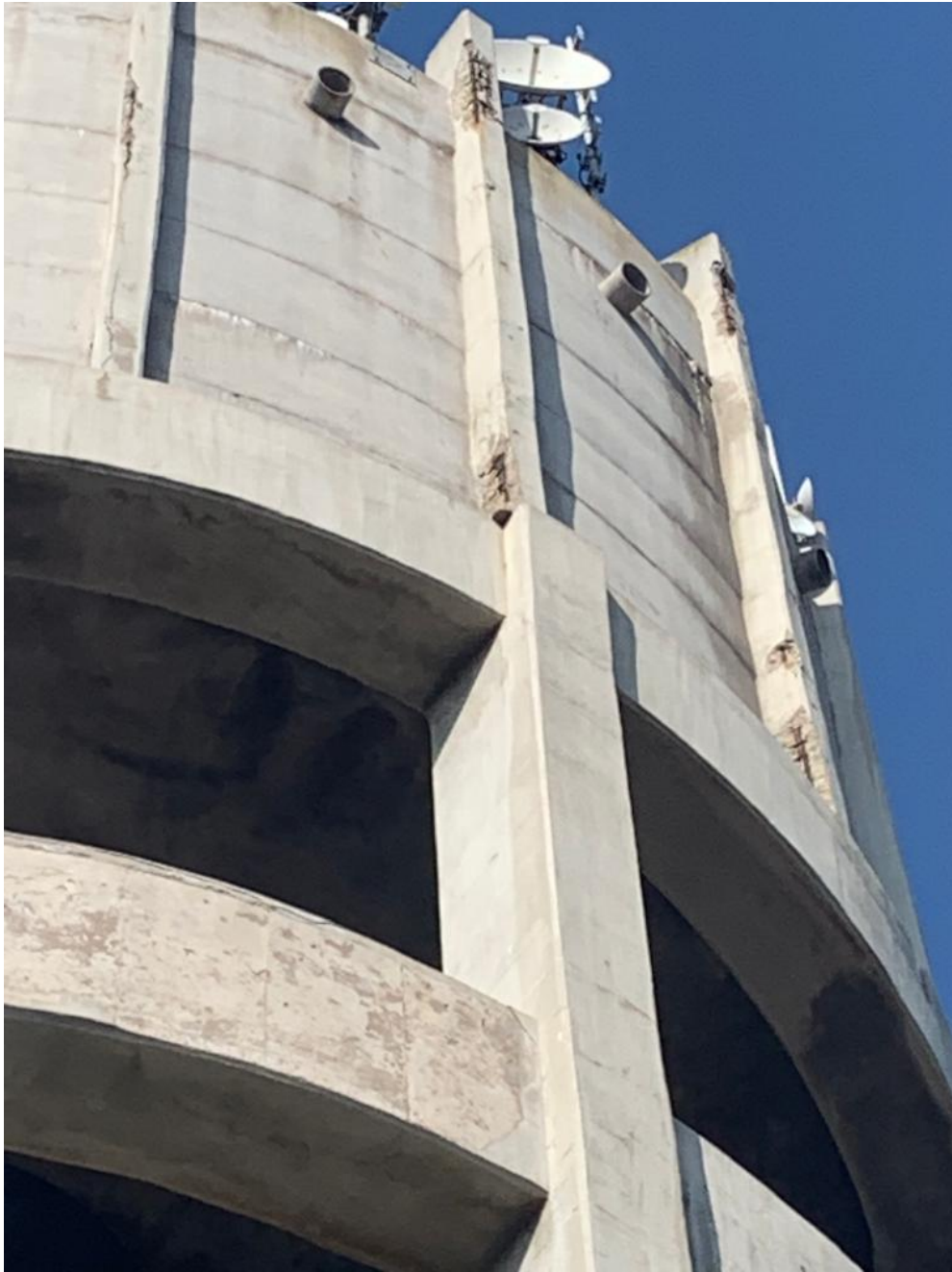
Figure 4: Paradise Beach Water Tower
