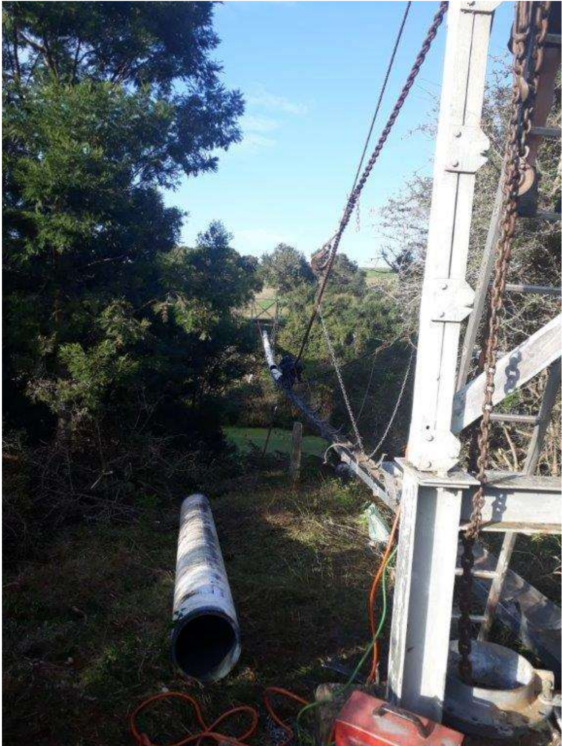
Figure 5: Repairs to Suspension bridge (2)
