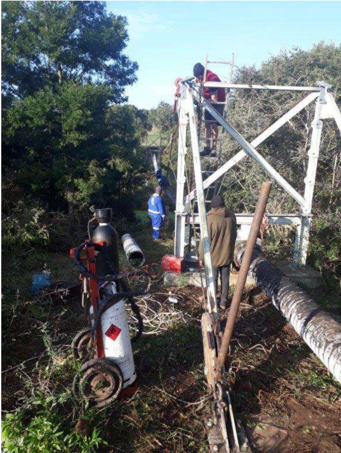
Figure 4: Repairs to Suspension Bridge
